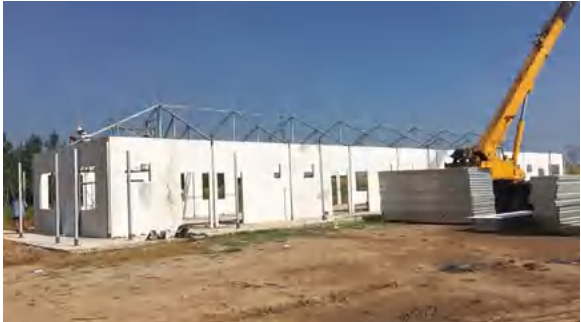
一体化外墙板安装 Integrated External Wallboard Installation
