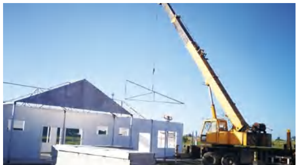
钢结构屋架吊装 Steel Roof Truss Lifting
